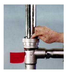
If reassembled correctly, the center of the ball indicator should lineup with the scale "zero" (either dotted black or scribed line). If it does not, disassemble the meter completely and carefully reassemble it, making sure the slotted meter tube is completely seated in the body.
